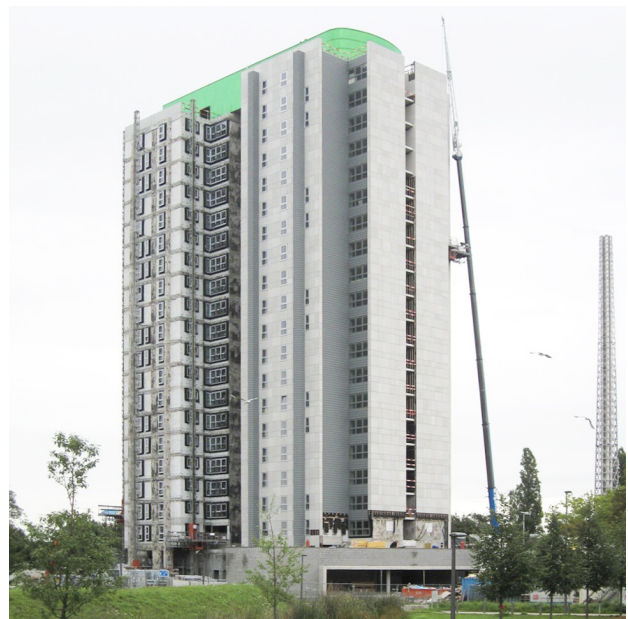
Kiel Silvertoren housing estate renovation (Antwerp)
